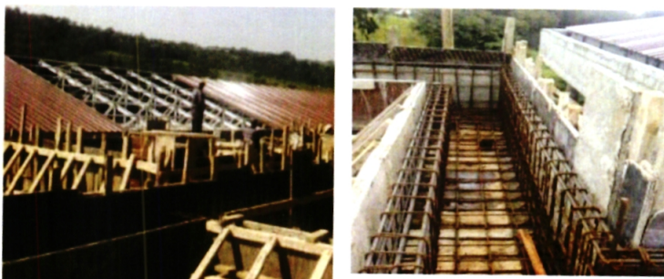
On-going Construction of Science Complex
