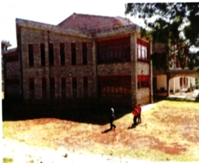
West side view of the Library Block
