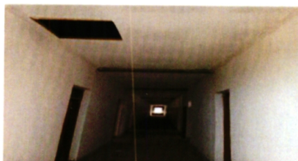
INTERIOR OF BLOCK A SCHEMING WORK
