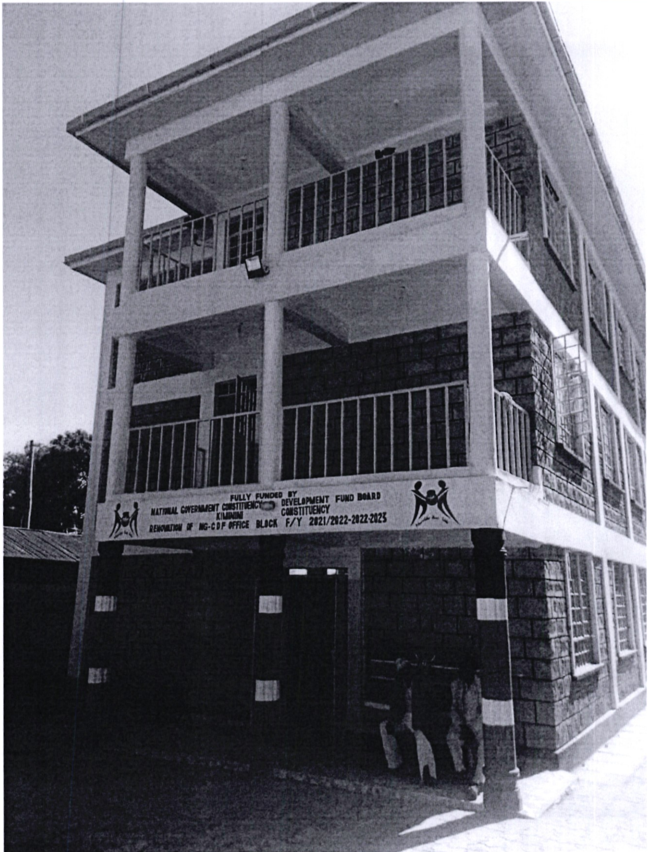
NG-CDF Kiminini Constituency Office- Construction of Office block, F/Y 2021-2022/2023
