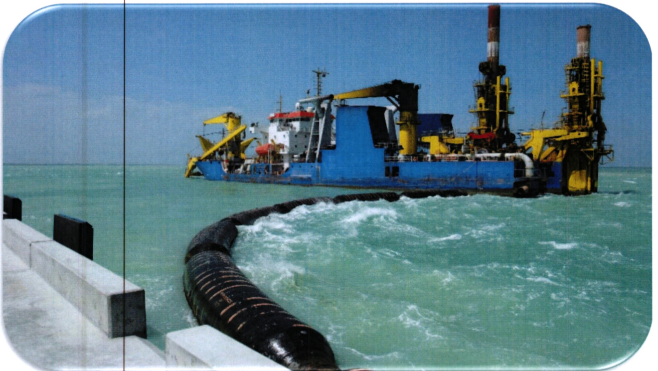
Figure 2: Dredging channels at the Port of Lamu
