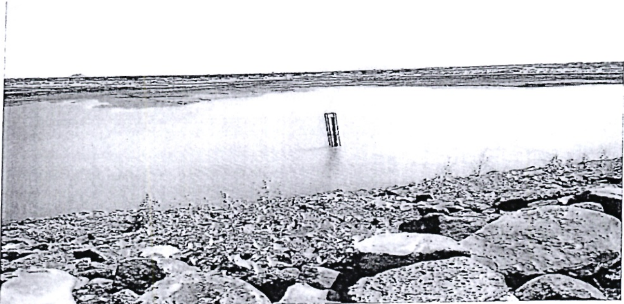
Idhido Dan- Volume of the embankment is 32,283 m 3
