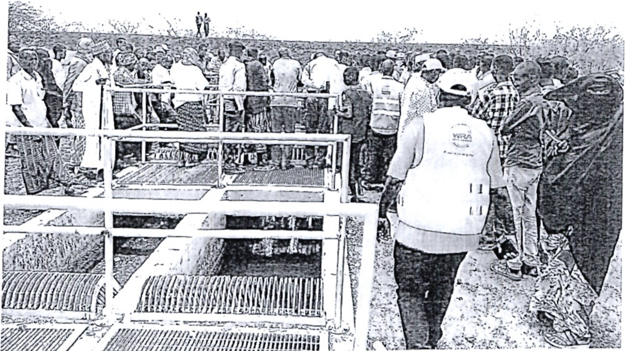
Principal Secretary of State Department of Water and Sanitation during Inspection tour at Garissa Sewerage Project- Inlet Works
