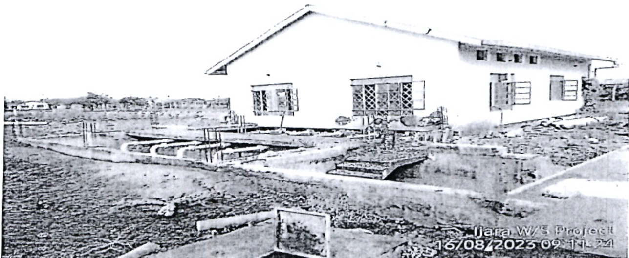
Masalani Ijara water supply-Pump house construction at intake works station
