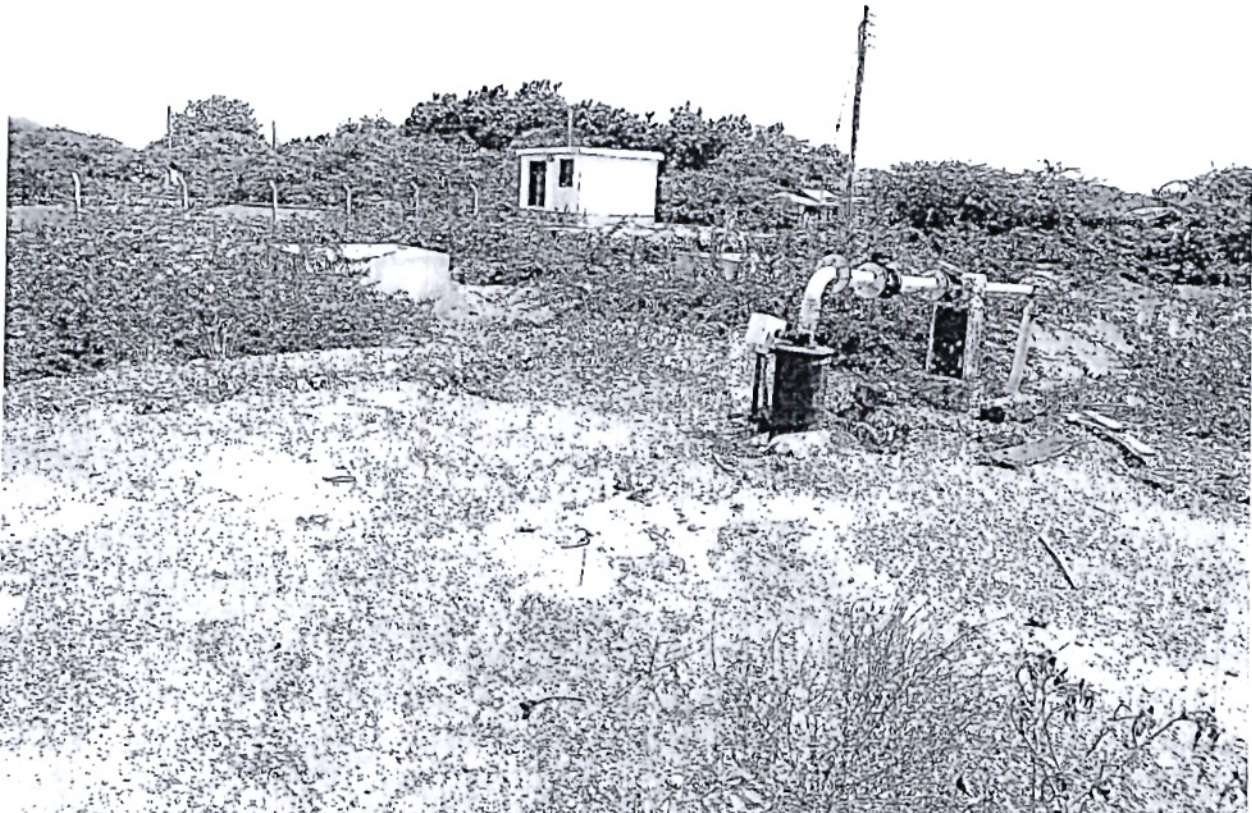
Last Mile connectivity Garissa-Borehole and power house
