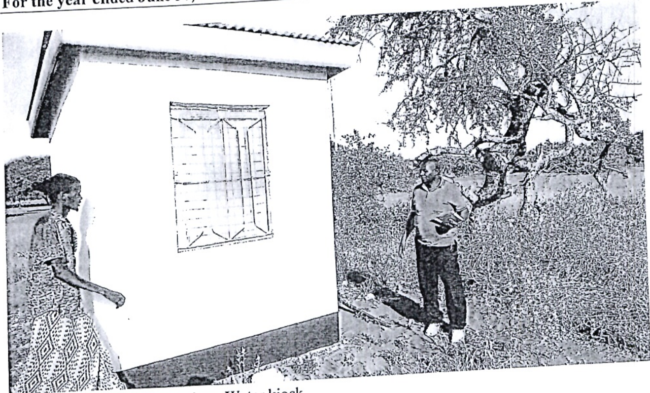
Bilatulamin Biad Water Project- Water kiosk
