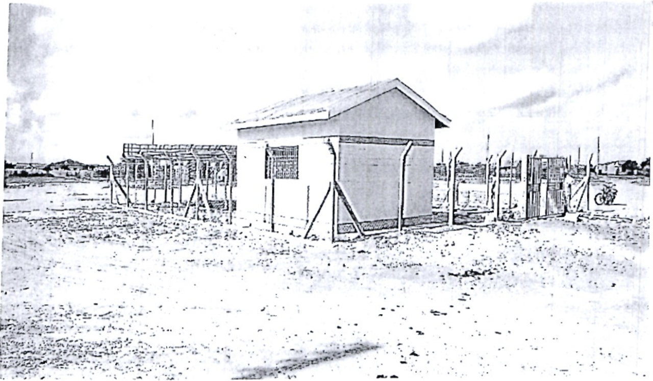
Habaswein Water Project-Pump House
