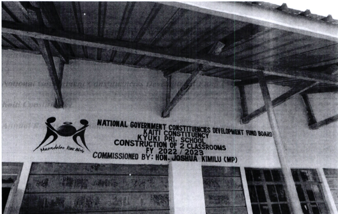
FIG 1: KYUKI PRIMARY SCHOOL-CONSTRUCTION OF 2 CLASSROOMS
