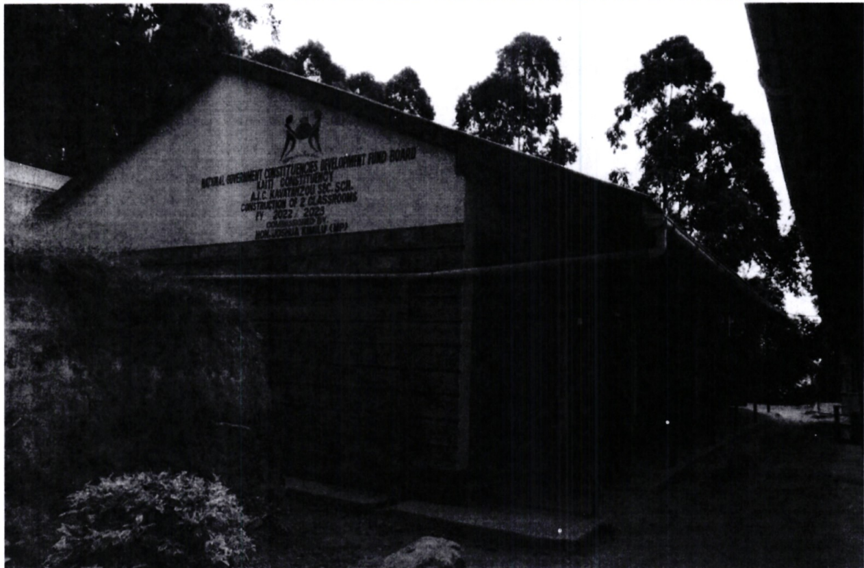
FIG 2: KAVATANZOU PRIMARY SCHOOL- CONSTRUCTION OF 2 CLASSROOMS
