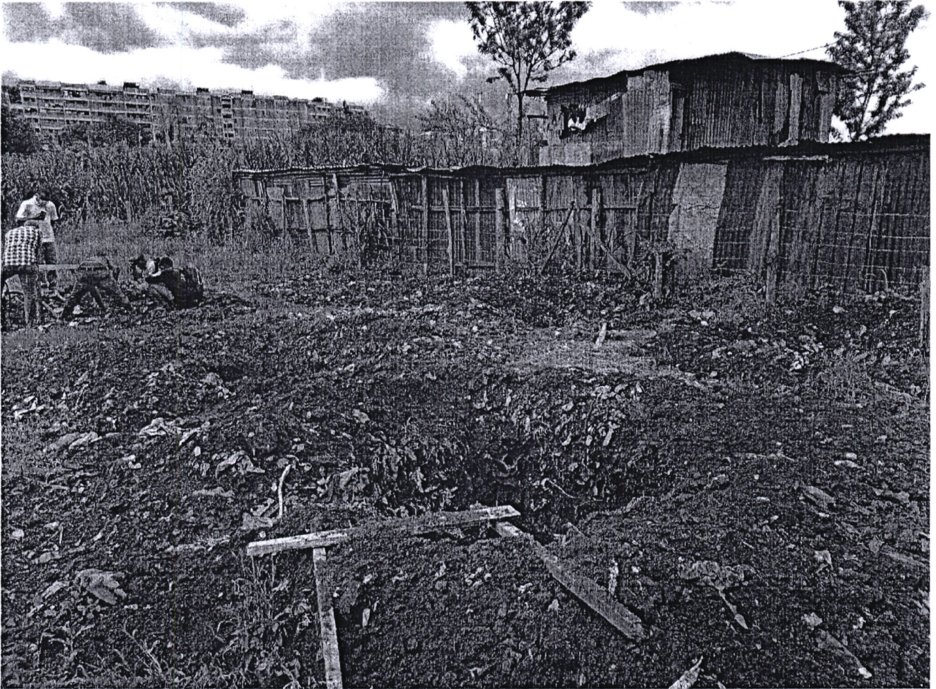
Joash Olum Highrise Primary School – Before the construction of a kitchen
