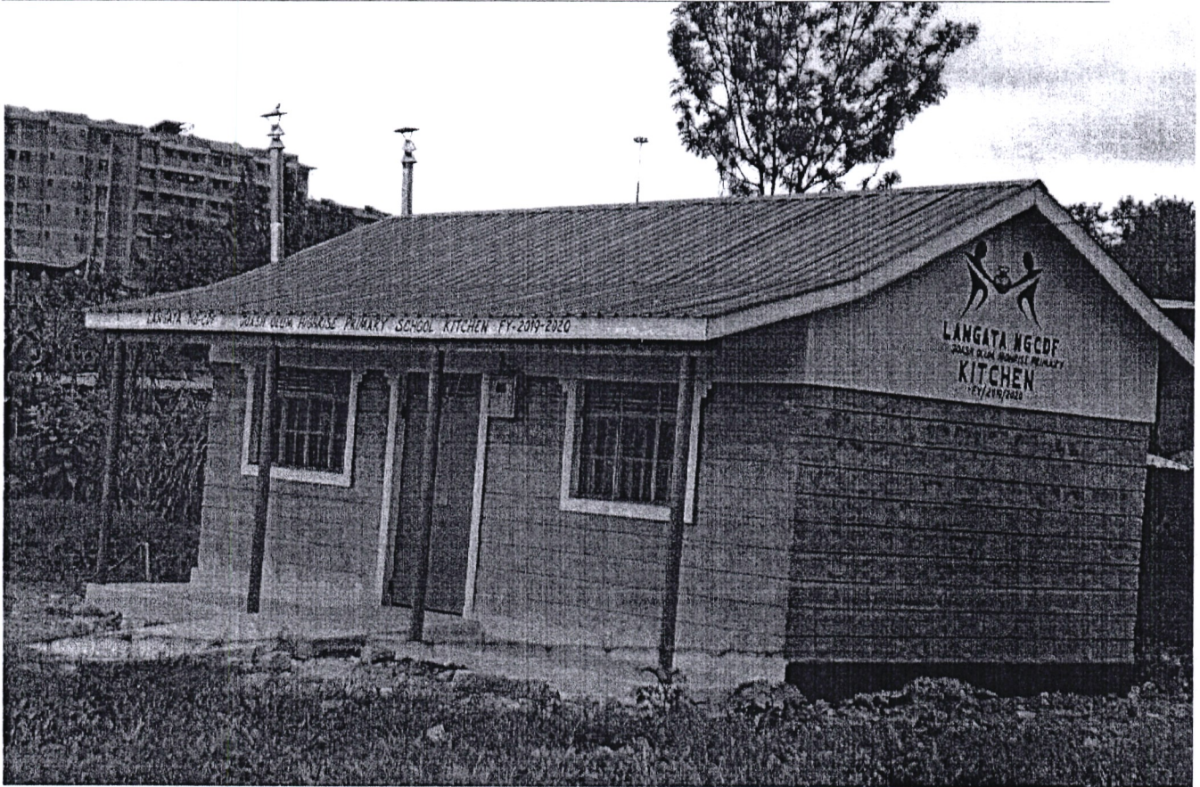
Joash Olum Highrise Primary School – After construction of a kitchen.
