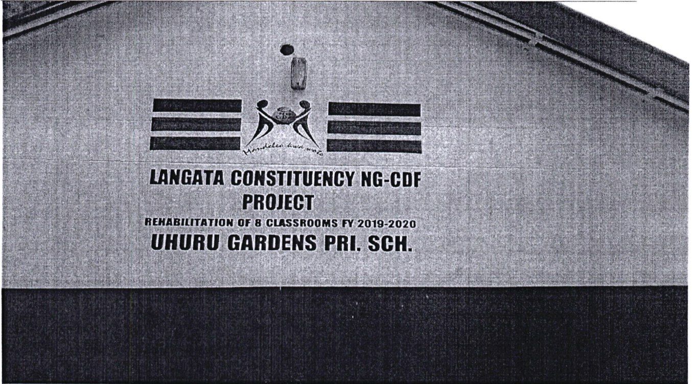
Uhuru Gardens Primary School – After renovation
