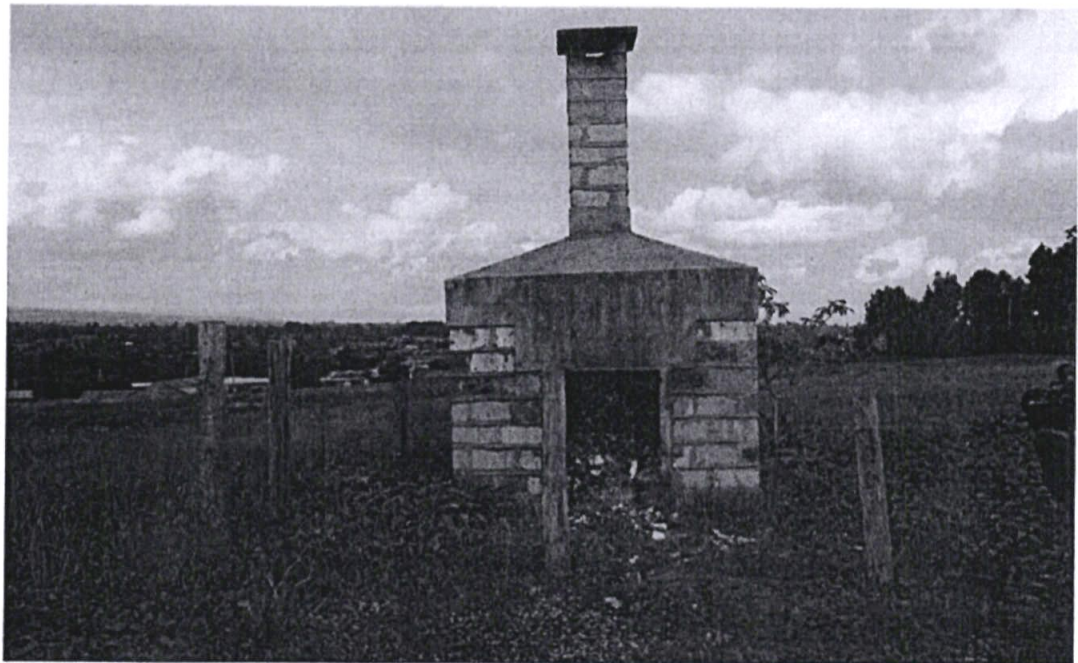
Picture 13: The committee observed that the hospital incinerator lacked a functional door and perimeter fencing, raising significant concerns regarding environmental safety.
