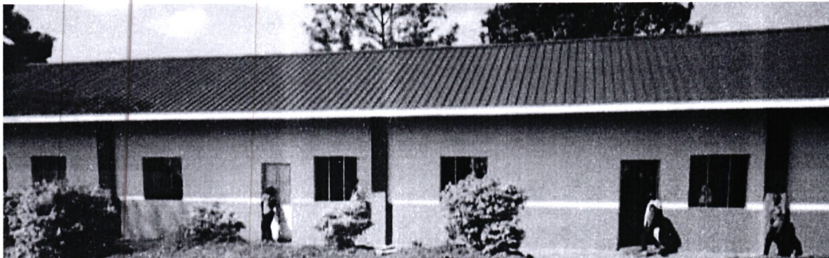
RENOVATED KIRERE PRIMARY SCHOOL CLASSROOMS
