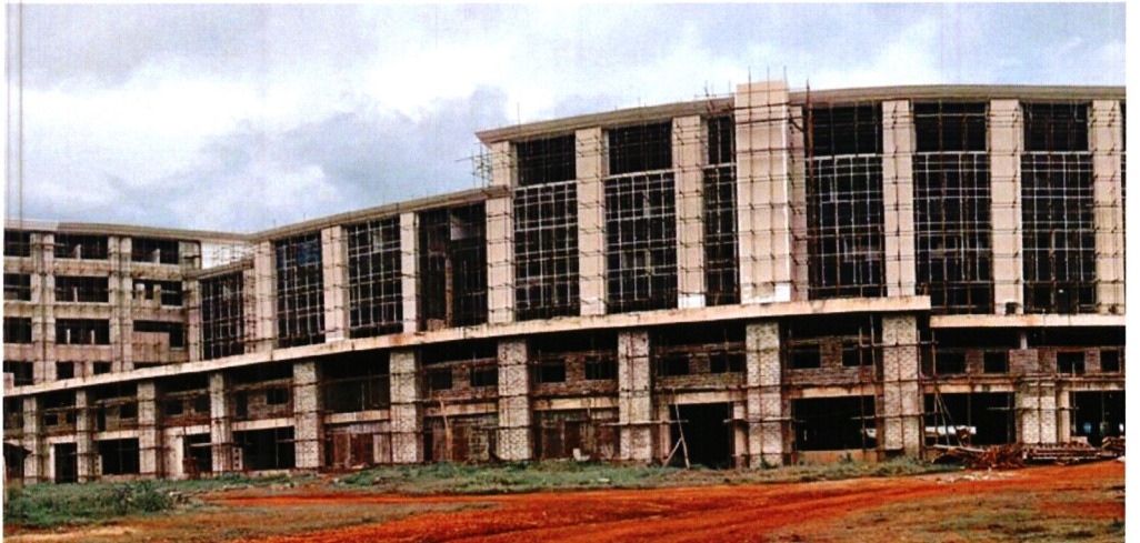
Kakamega Referral Hospital under construction 2019
