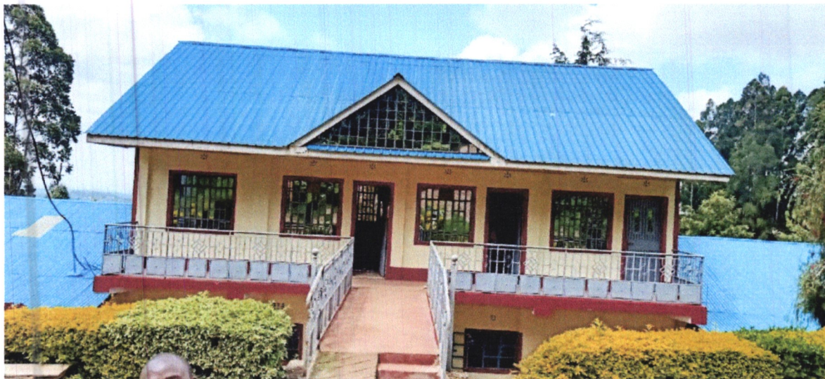
MUKUMU SECONDARY SCHOOL STOREYED COMPUTER LAB & CLASSROOMS BLOCK AT MURARANDIA WARD AFTER RENOVATION BY KIHARU NG-CDF
