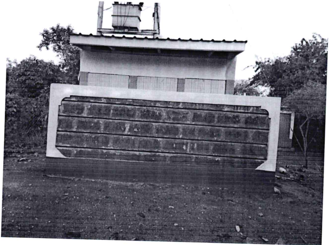
FIG 4: Ungatani Primary School-3 Door Pit Latrine
