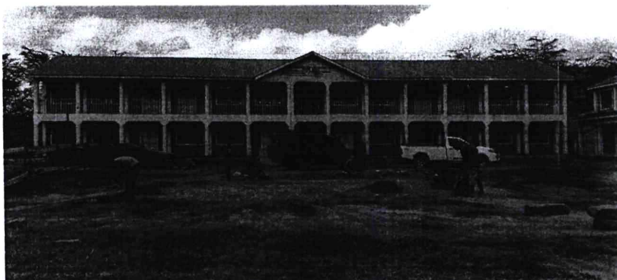
Storey tuition block of 8 classrooms
