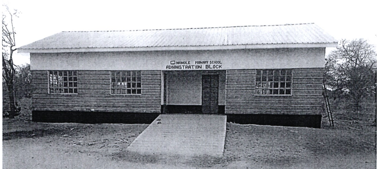
MAMOLE PRIMARY SCHOOL ADMINISTRATION BLOCK FROM FRONT VIEW
