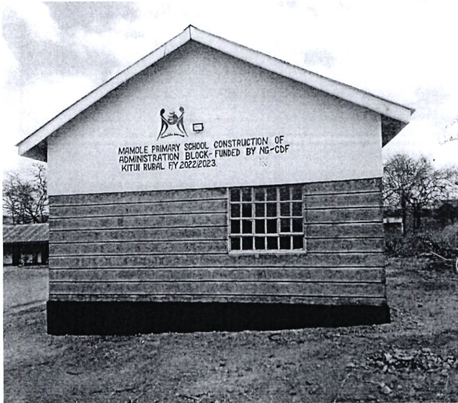
MAMOLE PRIMARY SCHOOL ADMINISTRATION BLOCK FROM THE SIDE VIEW
