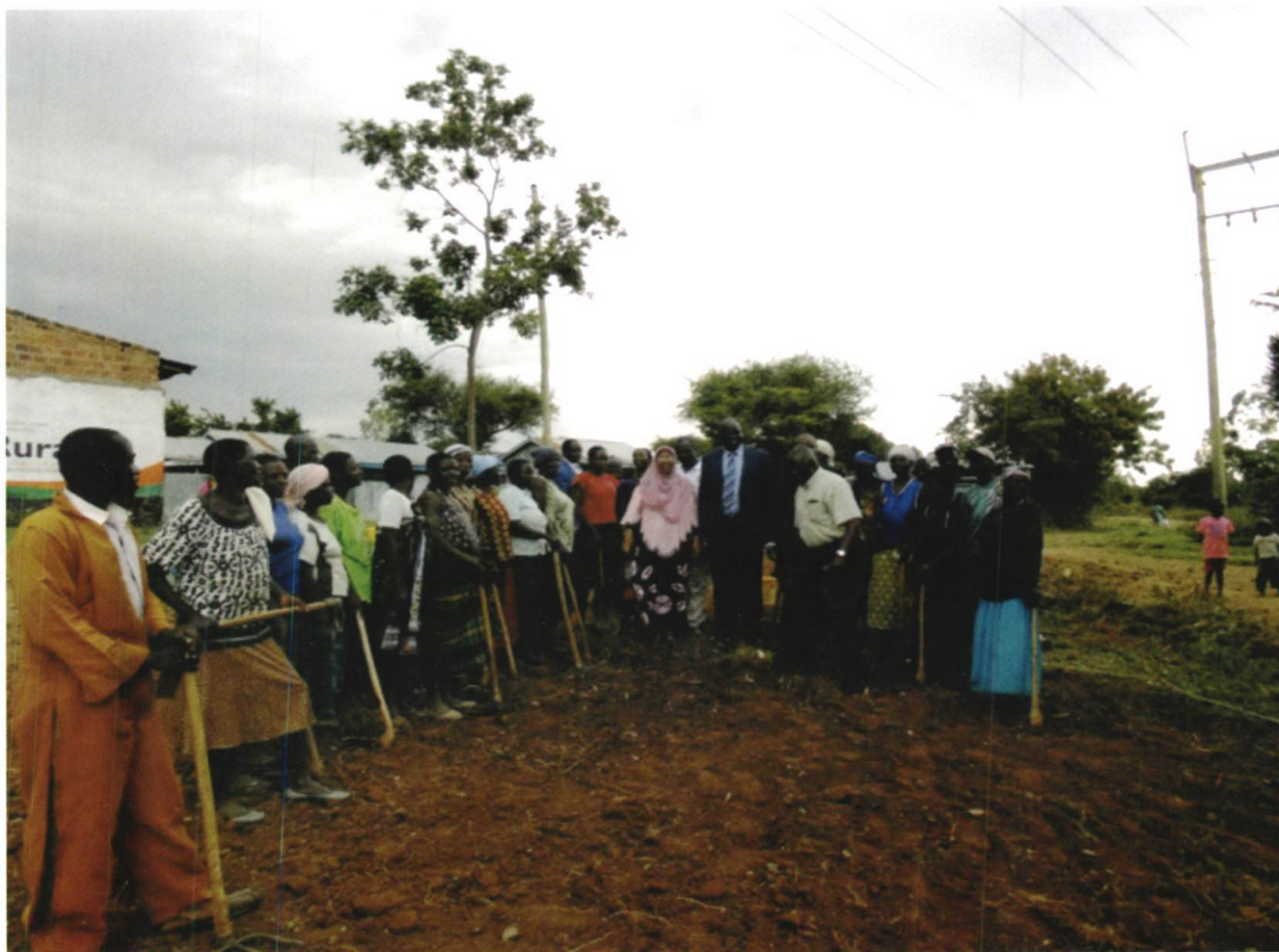
Fatuma Abdulkadir (front centre), Vice Chairperson CRA, together with members of the community from Homabay county who are constructing a road.
