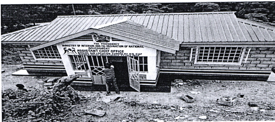
Sogon Chiefs Office -Construction Of Chiefs Office
