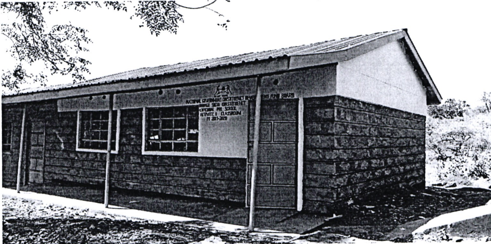
Kapkoibai Primary School – Construction Of 1 Classroom
