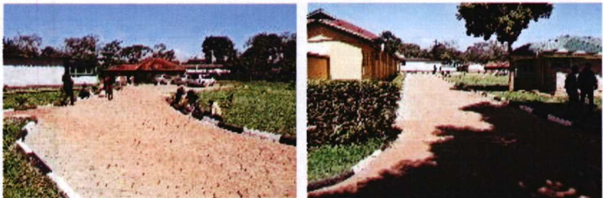
CONSTRUCTION OF ACCESS ROAD TO HOSPITALITY DEPARTMENT
