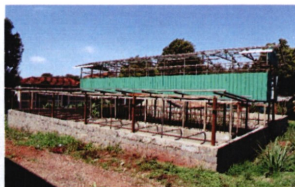
CONSTRUCTION OF DAIRY COWS SHED
