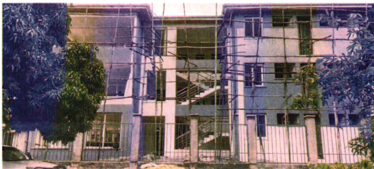
Ongoing construction of Machakos TSC County office
