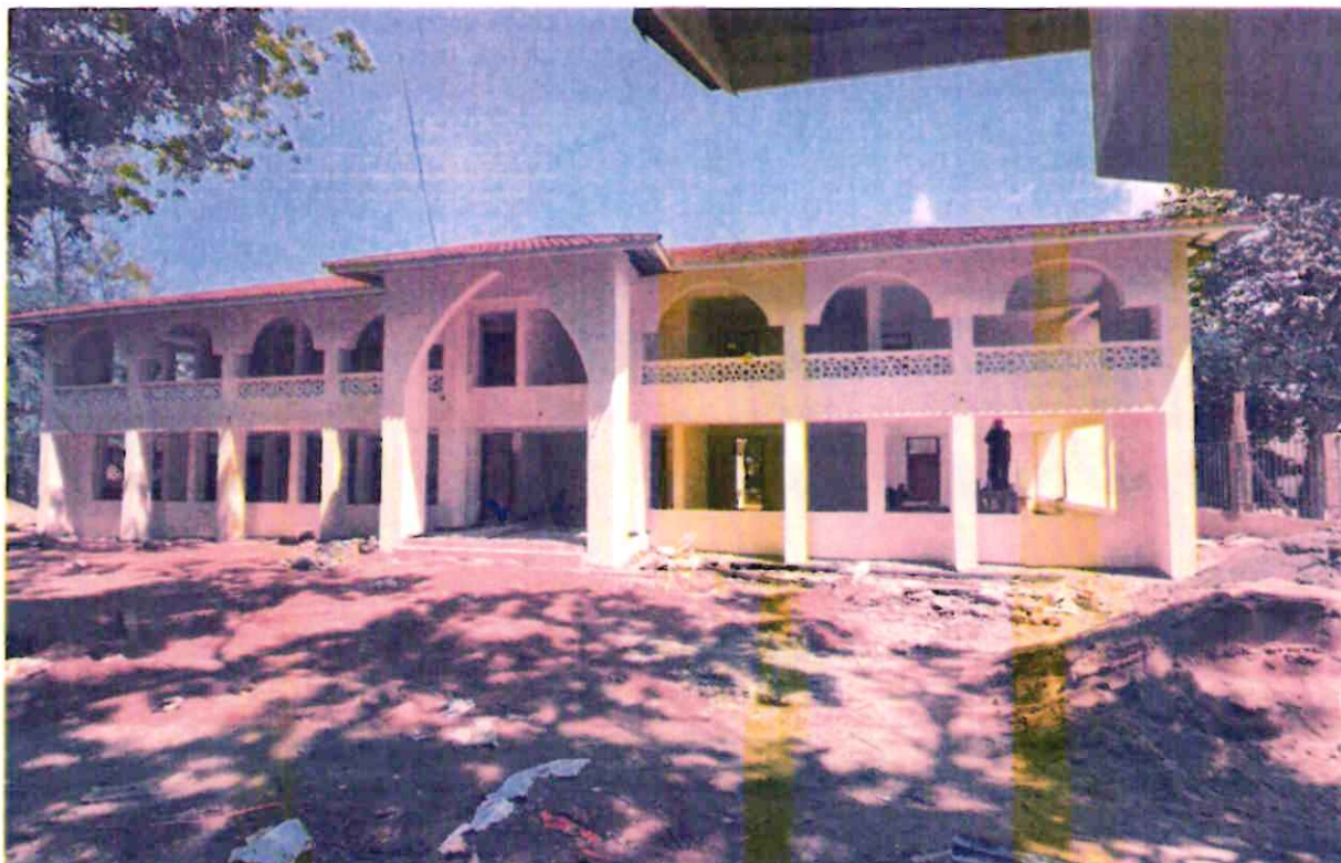
Ongoing construction of Kilifi TSC County office
