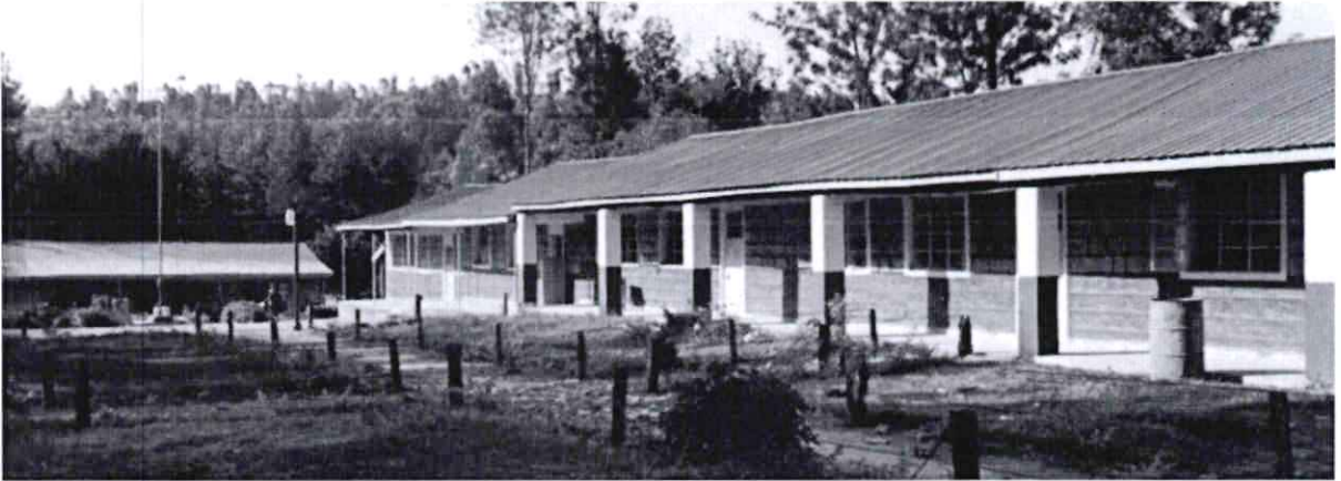
RENOVATION OF CLASSROOMS AT NGUTU PRIMARY SCHOOL
