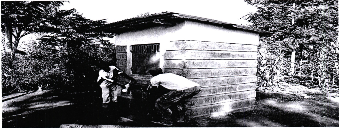
Figure 3: Mukindu Pry Sch borehole project.
