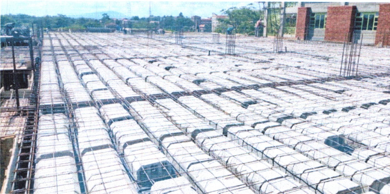
Slab construction - COETEC
