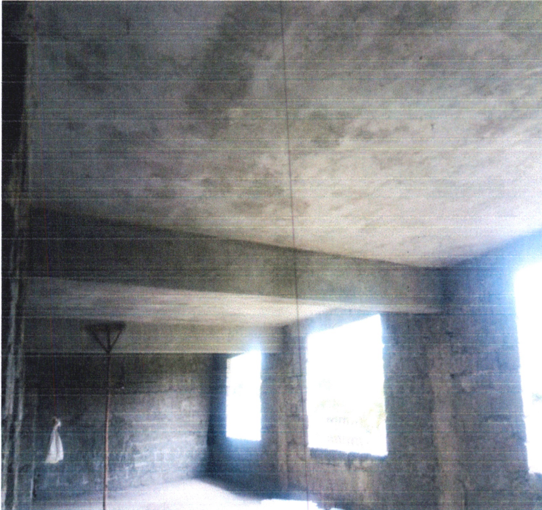
1 st floor ceiling plaster - COETEC
