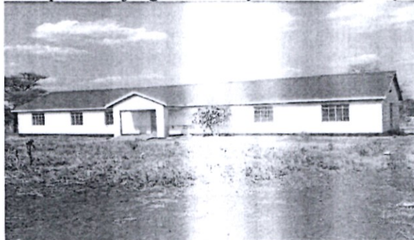
Bishop John Njenga secondary school dormitory
