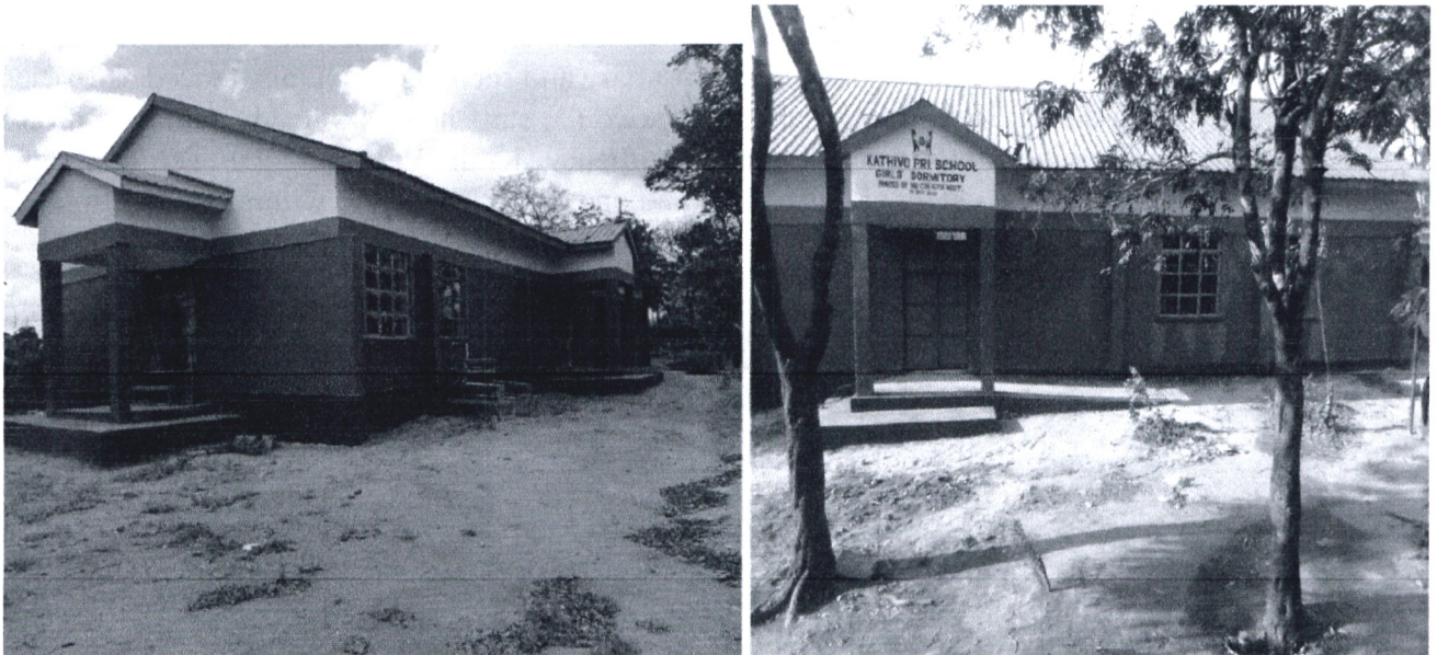
Figure 3: Construction of Dormitory at Kathivo Primary School
