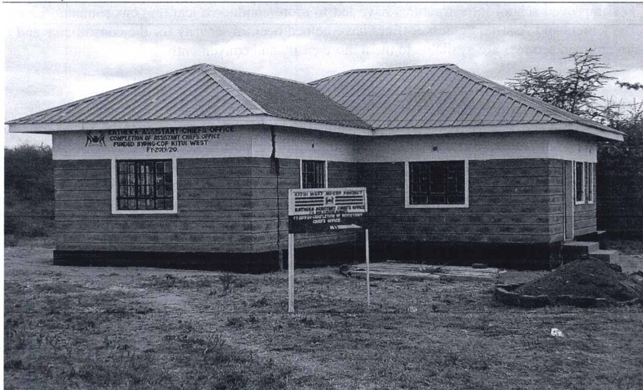
Figure 7: Completion of Katheka Assistant Chiefs Office
