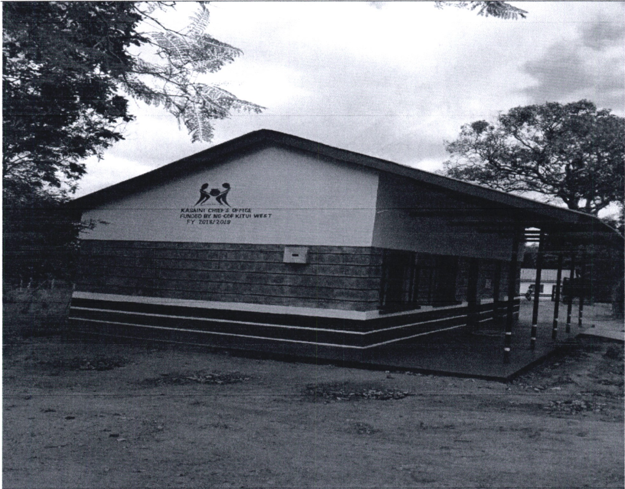
Figure 4: Construction of Kasaini Chiefs Office
