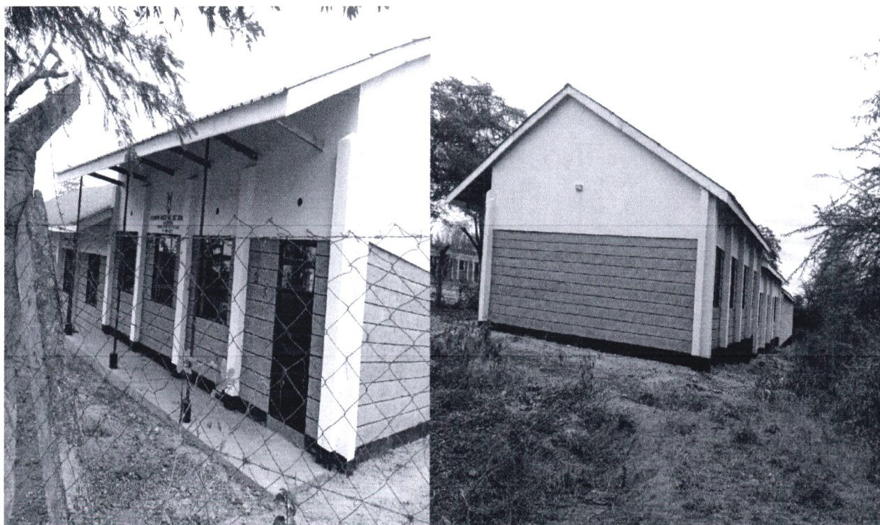
Figure 8: Construction of Three (3) classrooms at Kyondoni Mixed Day Sec. School
