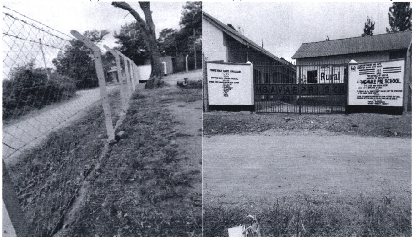
Figure 1: Fencing of Mbavae Primary School Compound.
