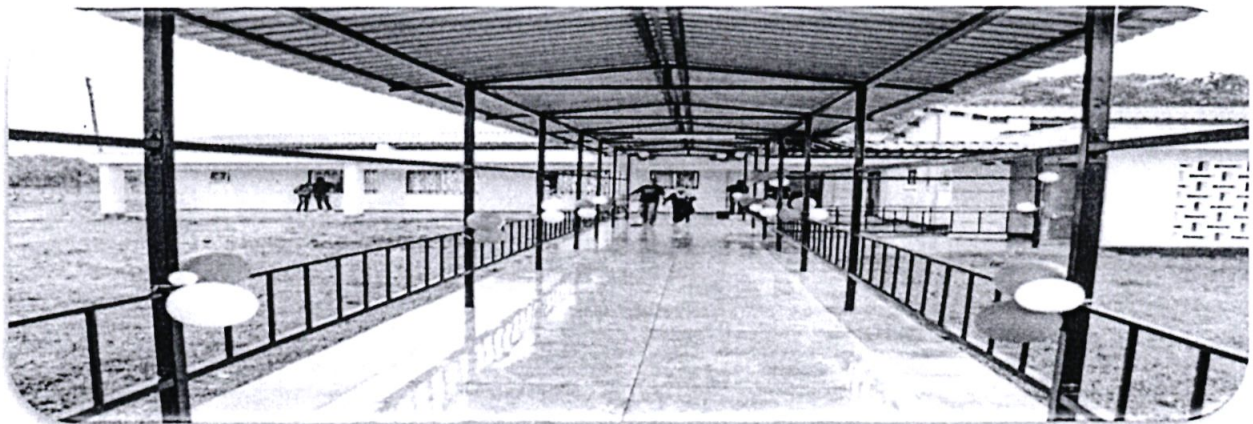
Figure 2: Picture of and upgraded section of the Mokowe Health Center
