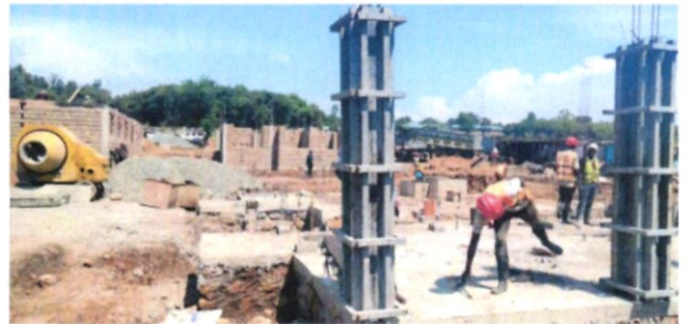
Work in progress at the Homa Bay AHP project
