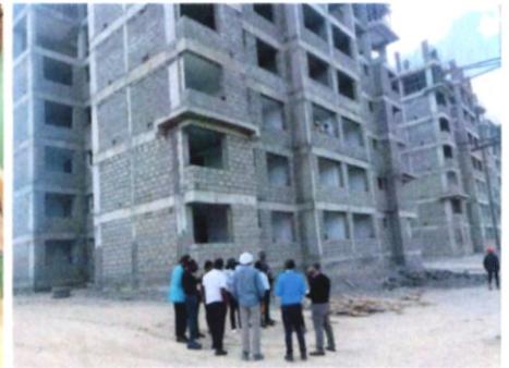
Stoni Athi Sector 2A project in Athi River, Machakos County
