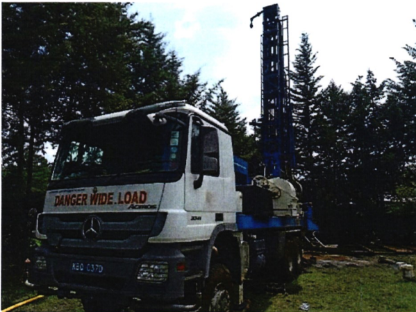
Drilling Community boreholes in Nyandarua County
