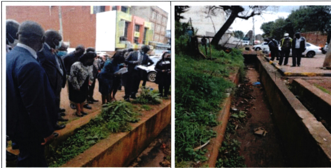
Figure 4: Construction of stormwater drainage facility-Kericho County
