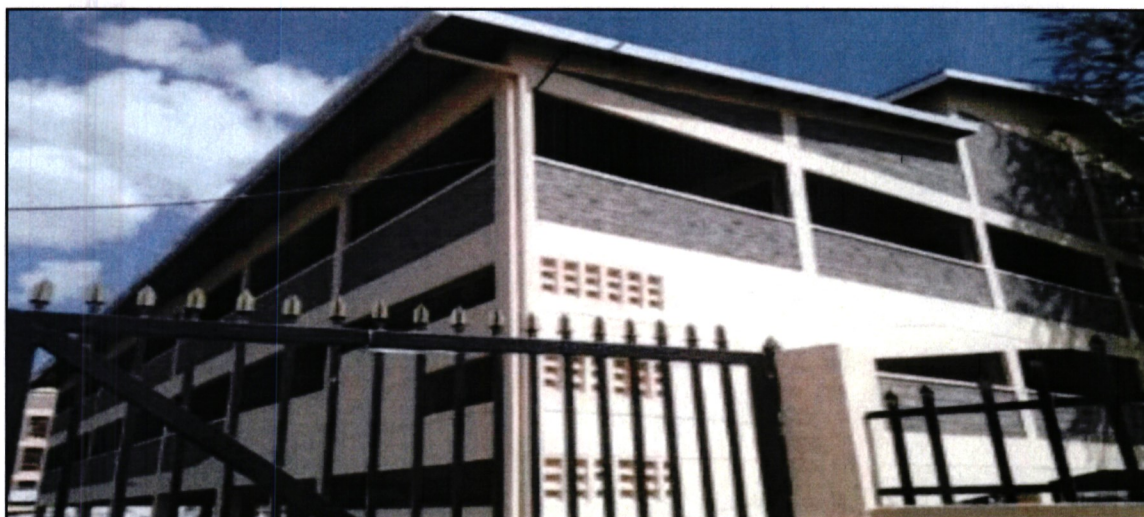
Figure 2: Construction of Kitengela Market-Kajiado County
