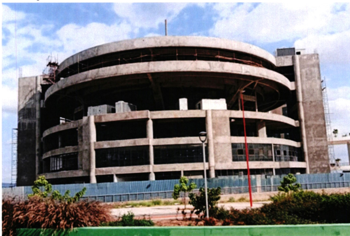
Conference Facility Superstructure Completion during the Financial Year
