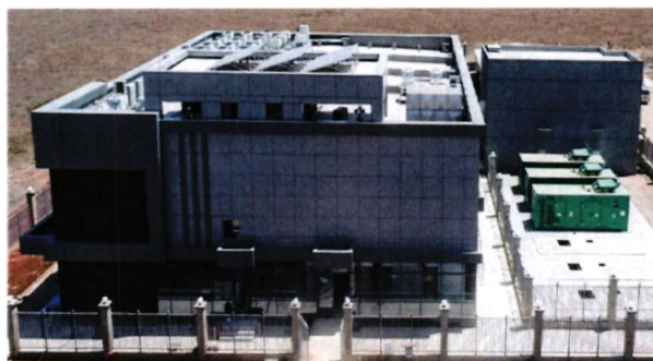
Phase 2 Data Centre
