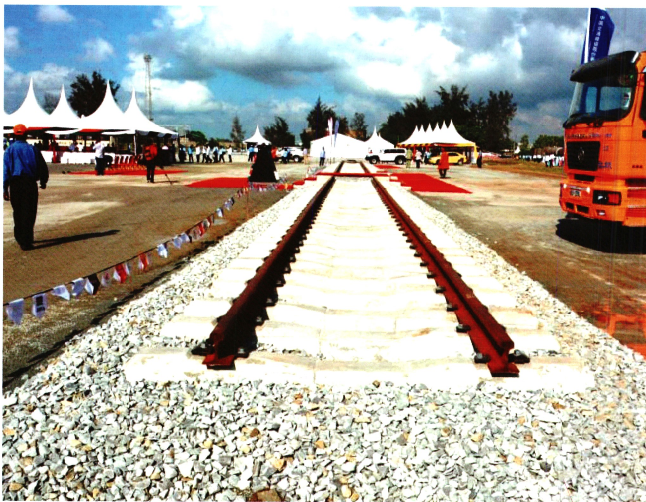
Laying of the standard gauge railway
