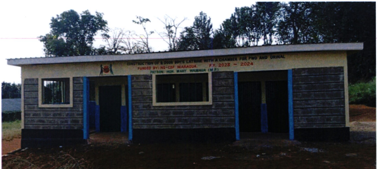
Igikiro primary school 8 door toilet block for girls
