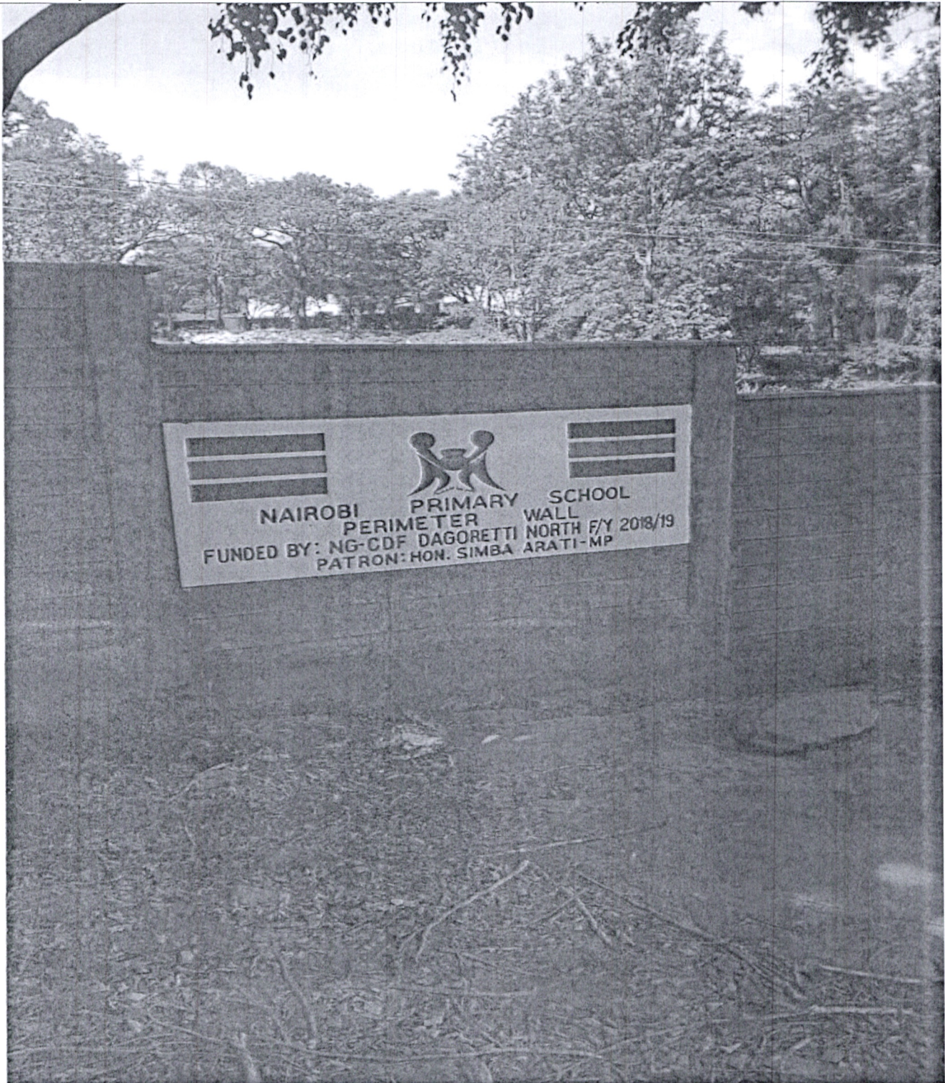
Figure 1: Construction of a Perimeter wall at Nairobi Primary School
