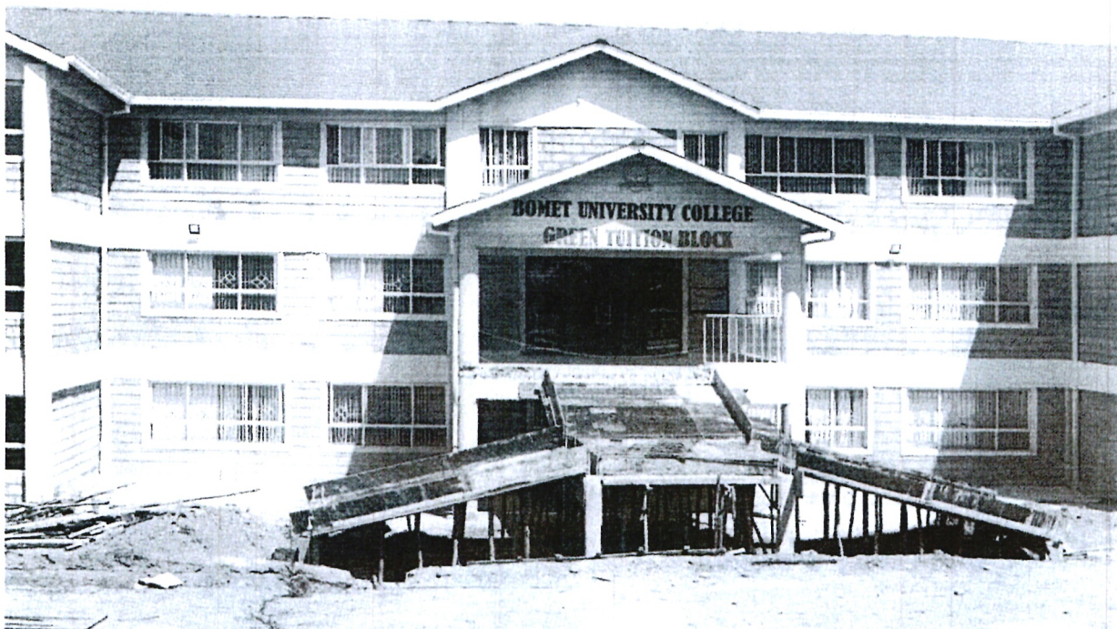
Picture 2: BUC Green Tuition Block- Front Elevation (99% completion) - Entry rum under construction.
