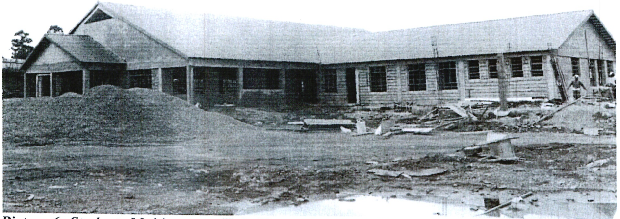
Picture 6: Students Multipurpose Hall (Front Elevation)- 60% completion
