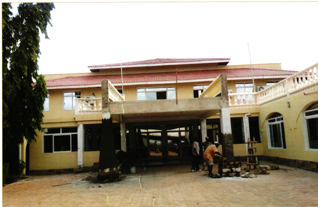
Kilifi Assembly Chambers under construction.
