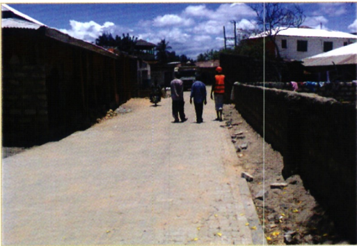
Watamu Township Cabro works.
