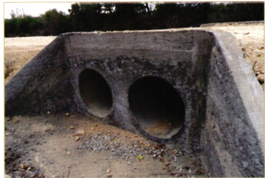
Marafa Chamari Road (culvert installation)
