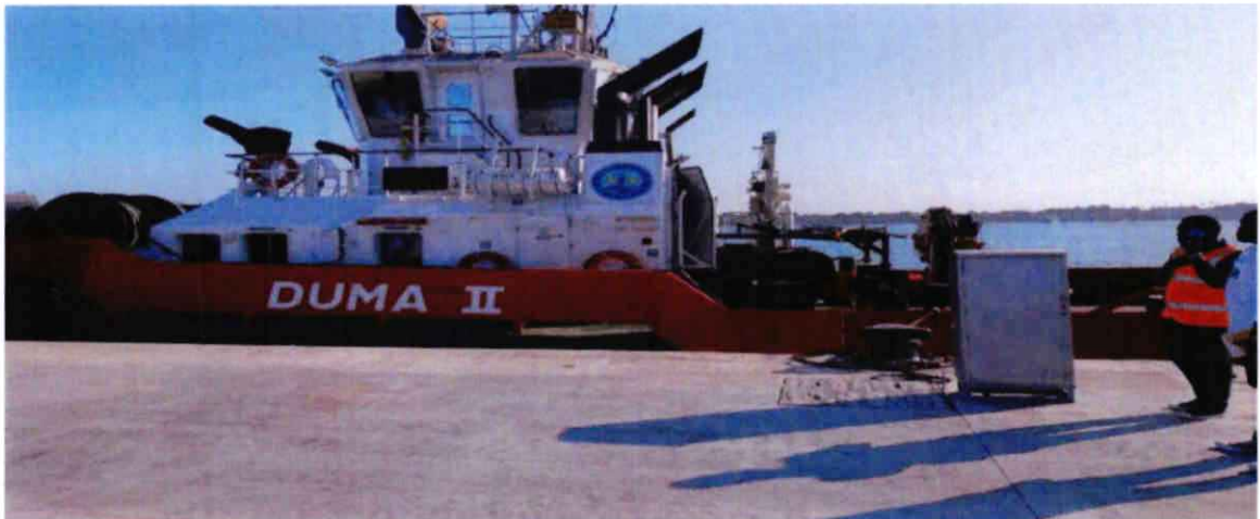
Tugboat jetty at dockyard fitted with shore power boxes
