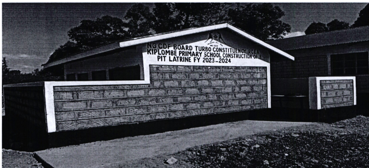
Kiplombe primary school pit latrine
