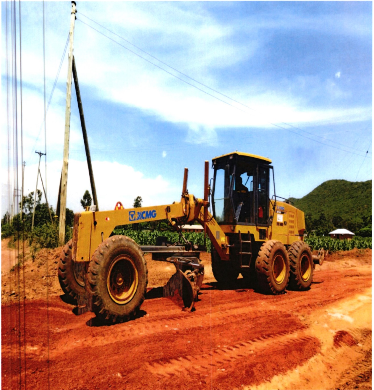
Road Grading Butula Constituency, Busia County.
