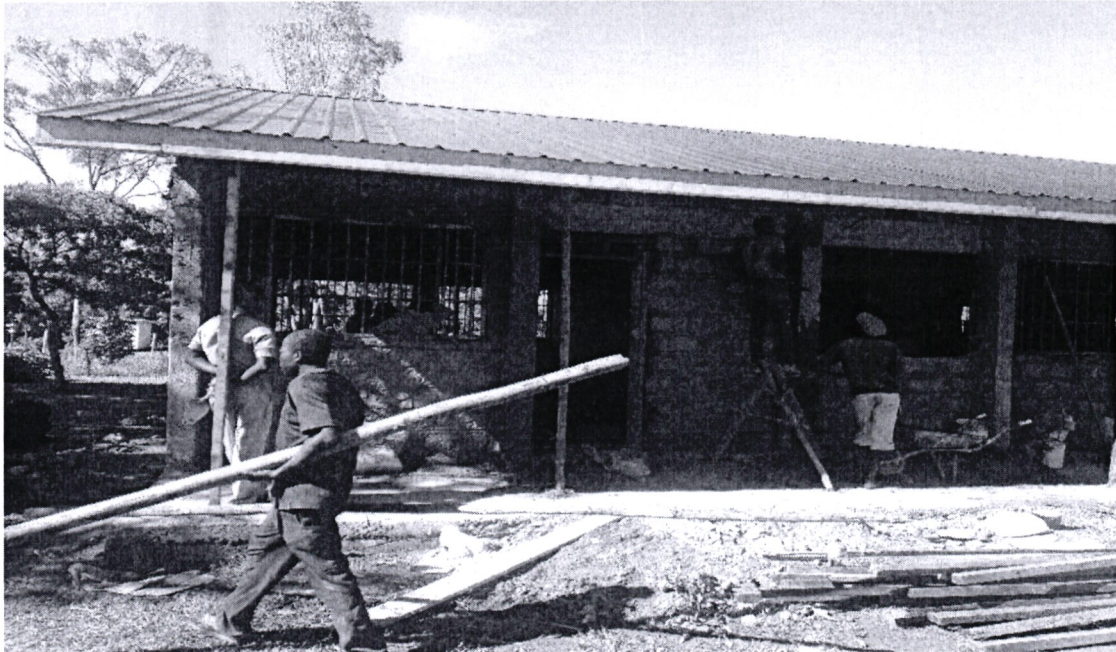
Ongoing construction works at Simbi Secondary School
