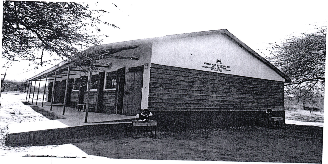
KAI PRIMARY SCHOOL-2 NEW CLASSROOMS CONSTRUCTED TO COMPLETION.
