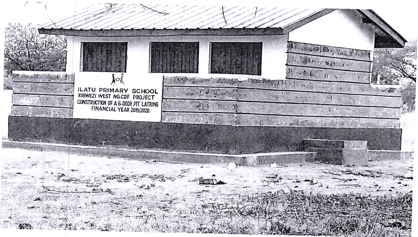
ILATU PRIMARY SCHOOL-Construction of 6doors pit latrines.
