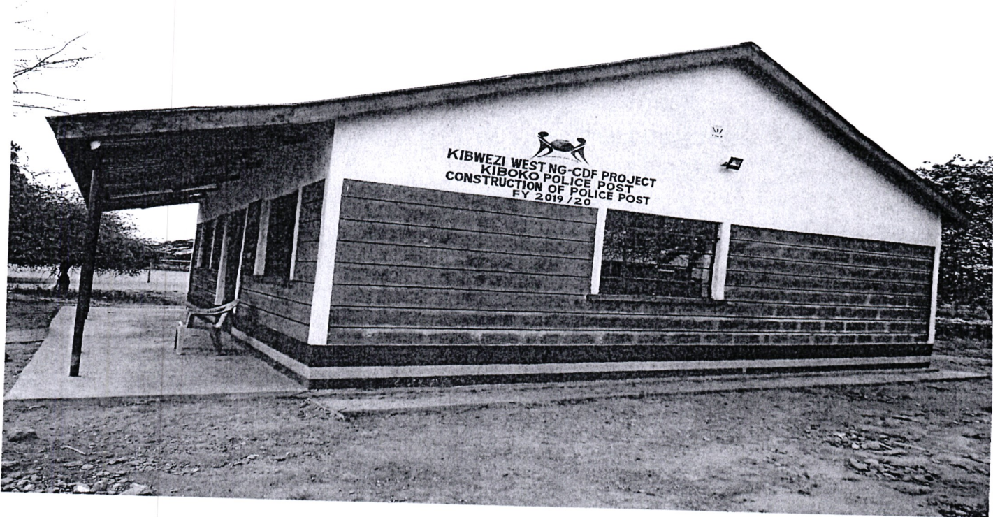
KIBOKO POLICE POST- Construction of a post with cell and armoury, supply of office table and chair and 10 plastic chairs.
