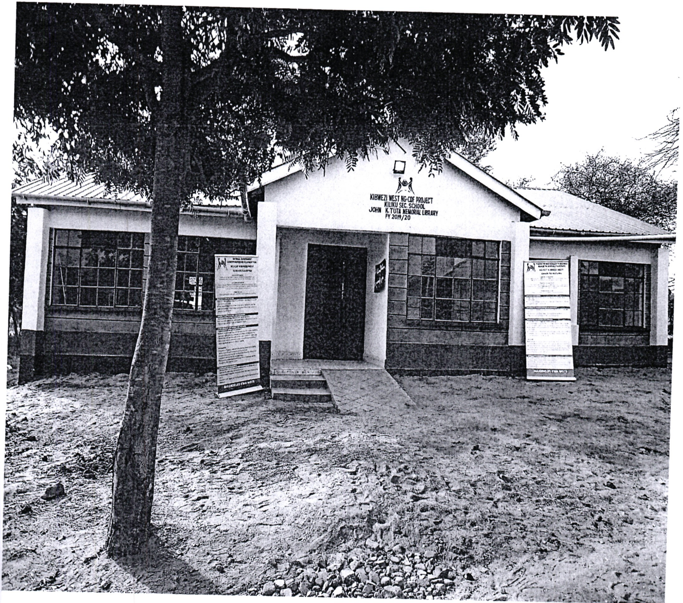
KILIKU MIXED SECONDARY SCHOOL.-Construction of library and provision of book shelves.
