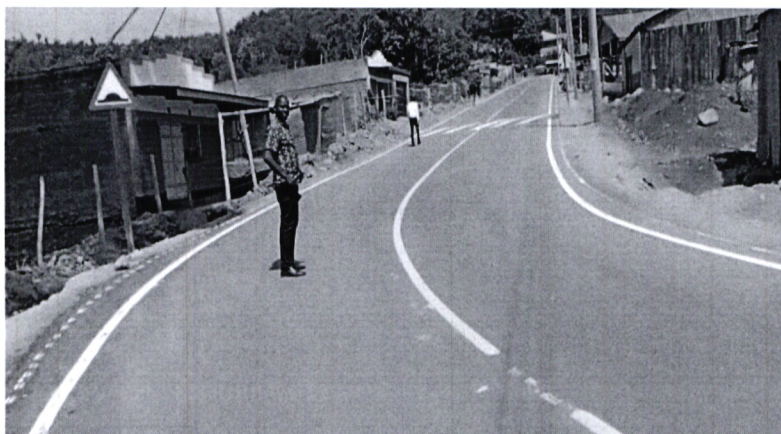
Longisa Road markings and road signage
