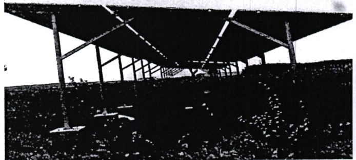
Solar panel array in Alupe
