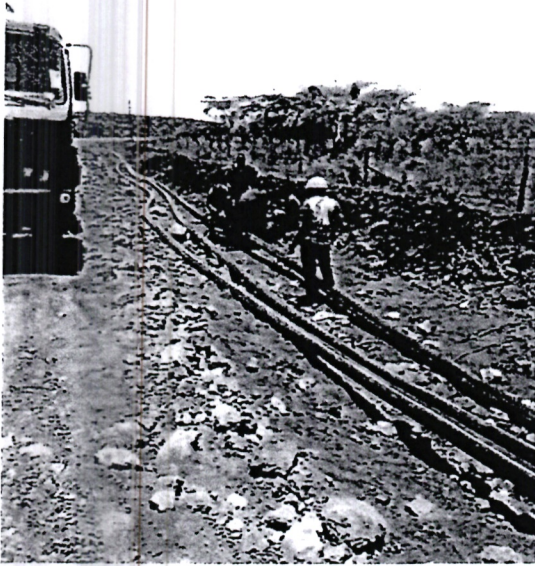
Excavation for laying of the 17 km pipel 1
