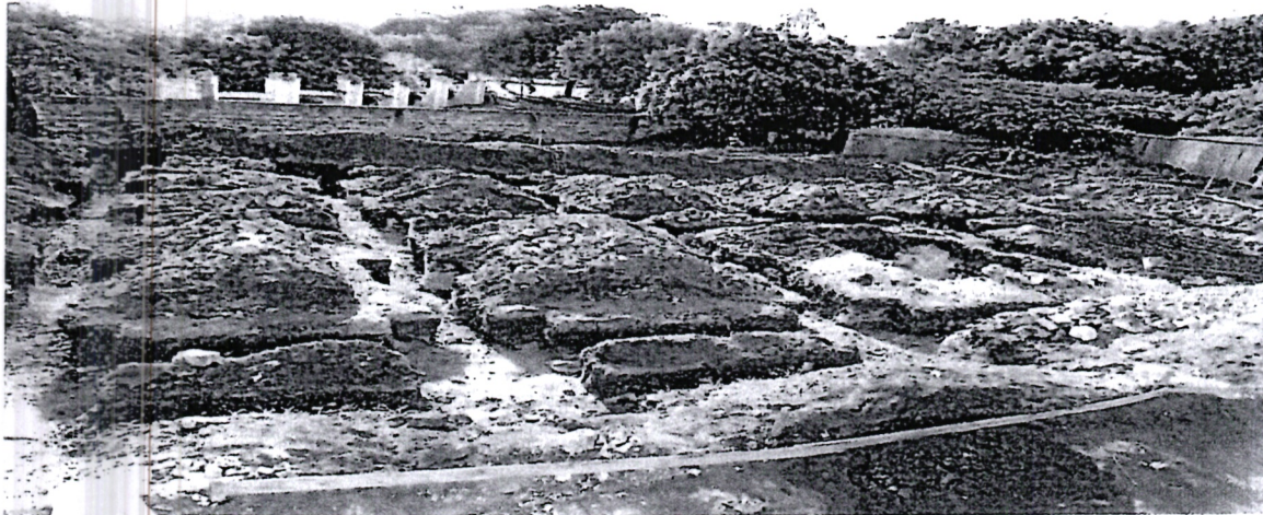
Figure 50: Foundation of the new accommodation rooms
