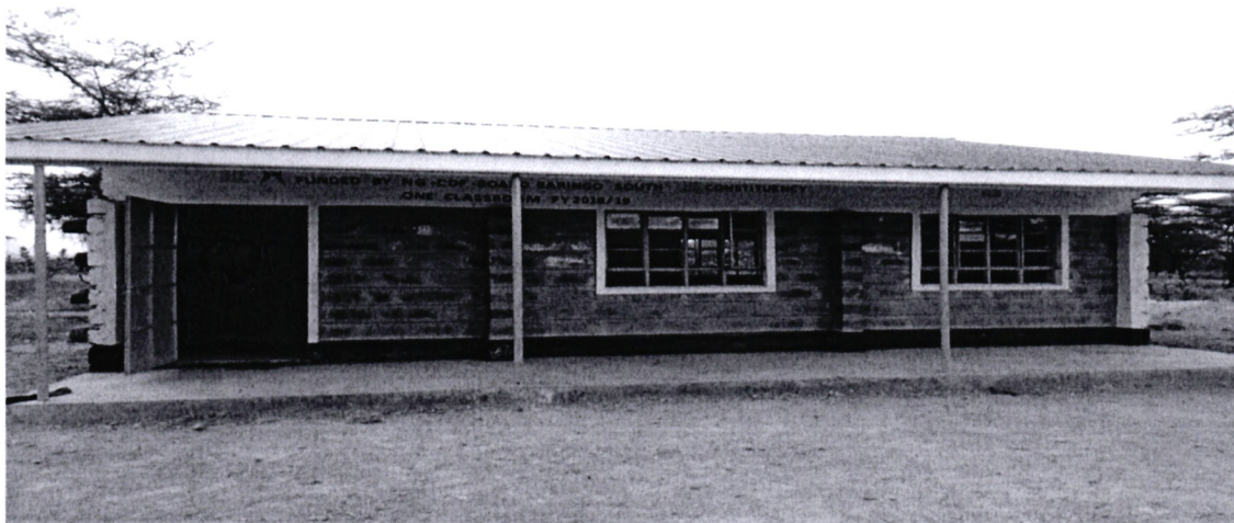
KIMAO PRIMARY SCHOOL – CONSTRUCTION OF 1 CLASSROOM
