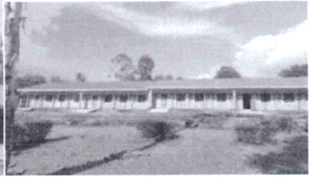
4 classrooms constructed at ombo primary school
