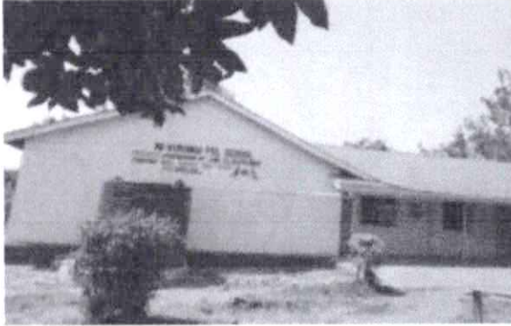
Renovation of st Thomas wikongaro Primary school.
