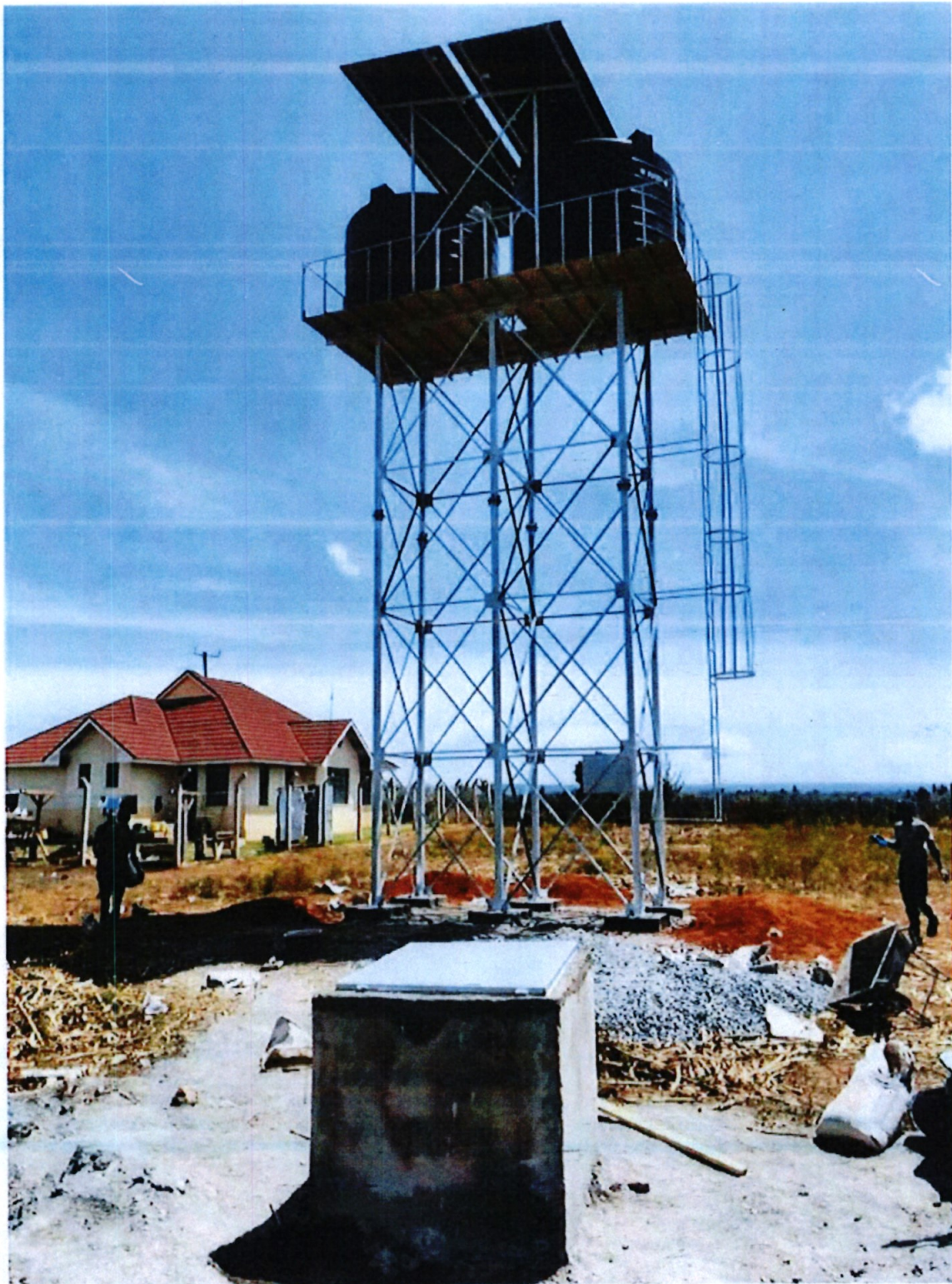
Figure 2 Borehole at Kelvin Kiptums home in Uasin Gishu
