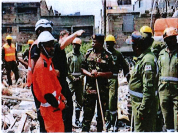
Figure 3 Kahawa West Building Collapse
