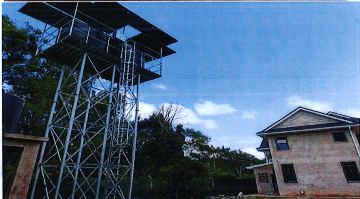
Figure 1 Kakuyuni HCA Borehole Machakos County
