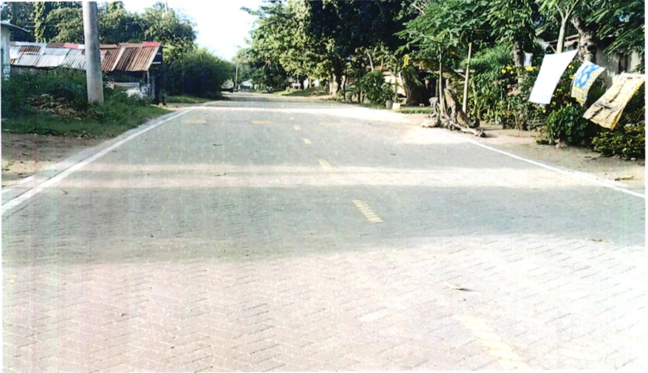
Cabro paving of Kombani Kwa Chief to Mtsangatifu road
