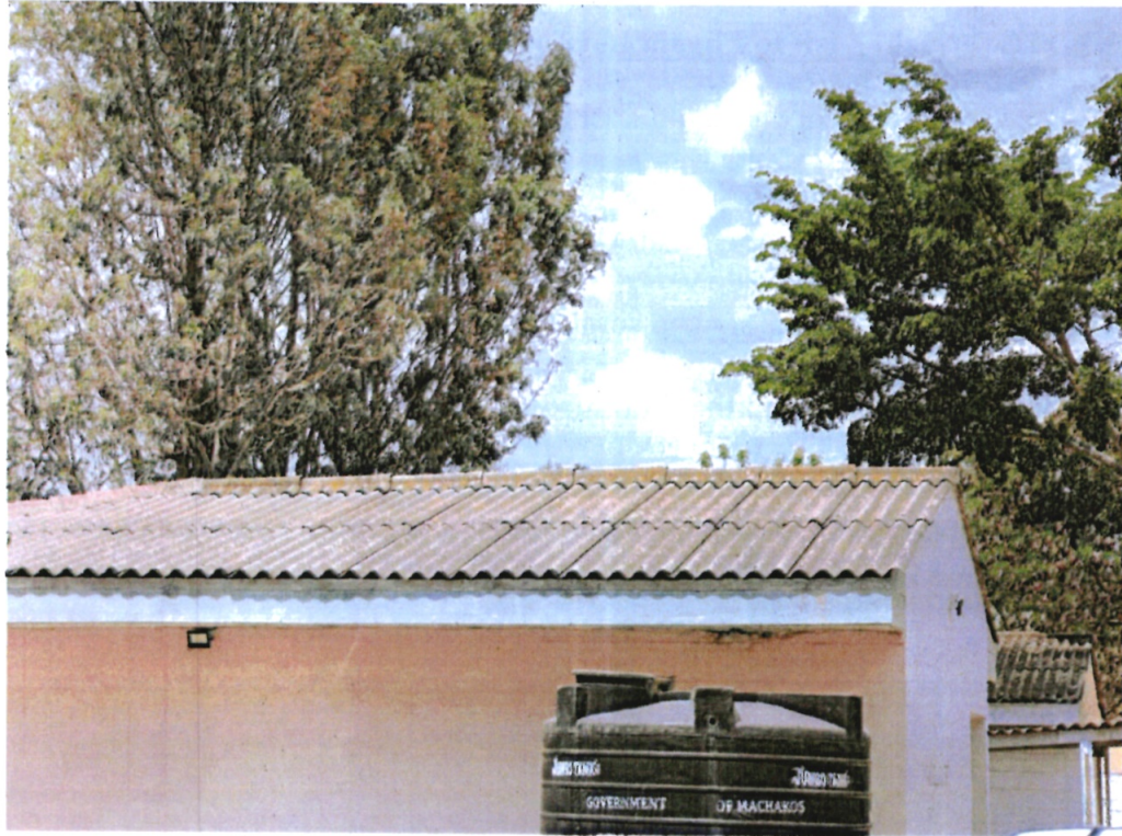
Picture 27: A roof with asbestos at the Mwala Level 4 Hospital which is scheduled to be removed and disposed before the end of the 2024/2025 Financial Year.
