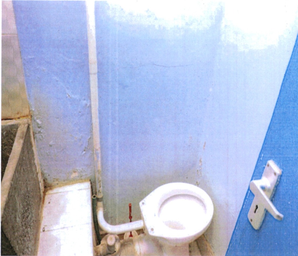
Picture 9: The bathrooms at the Hospital were dilapidated with visible cracks, peeling paints on the wall and signs of prolonged water damage on the walls and floor suggesting poor maintainance.
