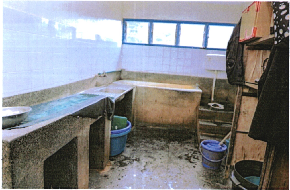
Picture 3: The renal washing area was in a deplorable state, characterized by dirt accumulation, old and rusty washing sinks and corroded surfaces.
