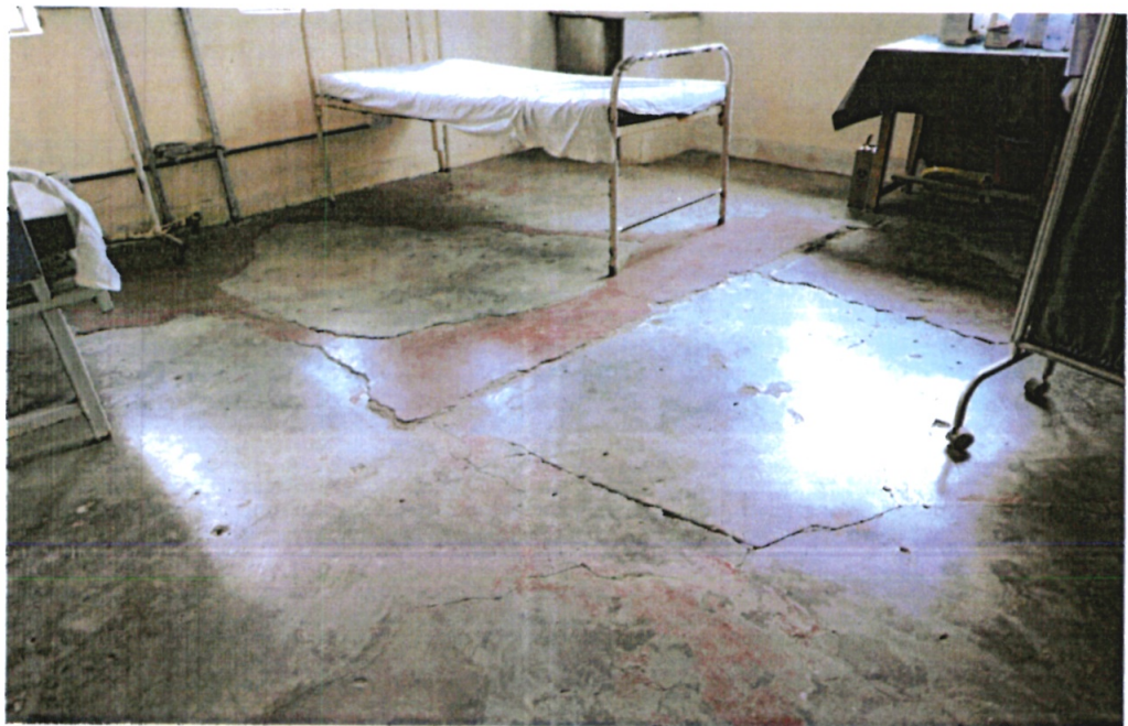
Picture 22: A Ward at the Athi River Level 4 Hospital face with poor physical infrastructure conditions including cracked floors.
