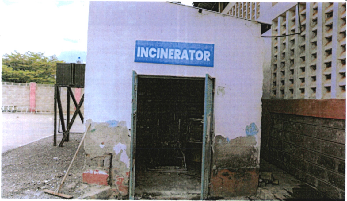
Picture 30: The incinerator at Machakos County Referral Hospital which does not have a functional entrance door.
