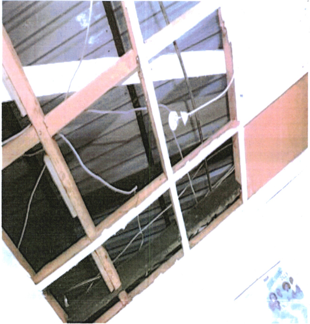
Picture 8: The section of the ceiling at Kitui Referral Hospital which had fallen off and ceiling panels are missing, exposing the internal framework, wooden beams, electrical wiring and the underlying metal roofing sheets.
