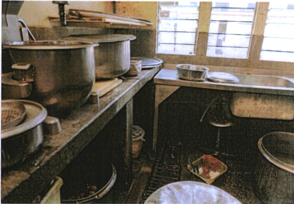
Picture 18: The Kitchen had rusty sinks, chipped walls, damaged work surfaces.
