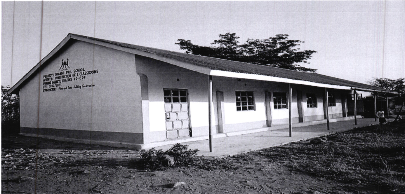
Construction of 2 classrooms at Orango Primary school
