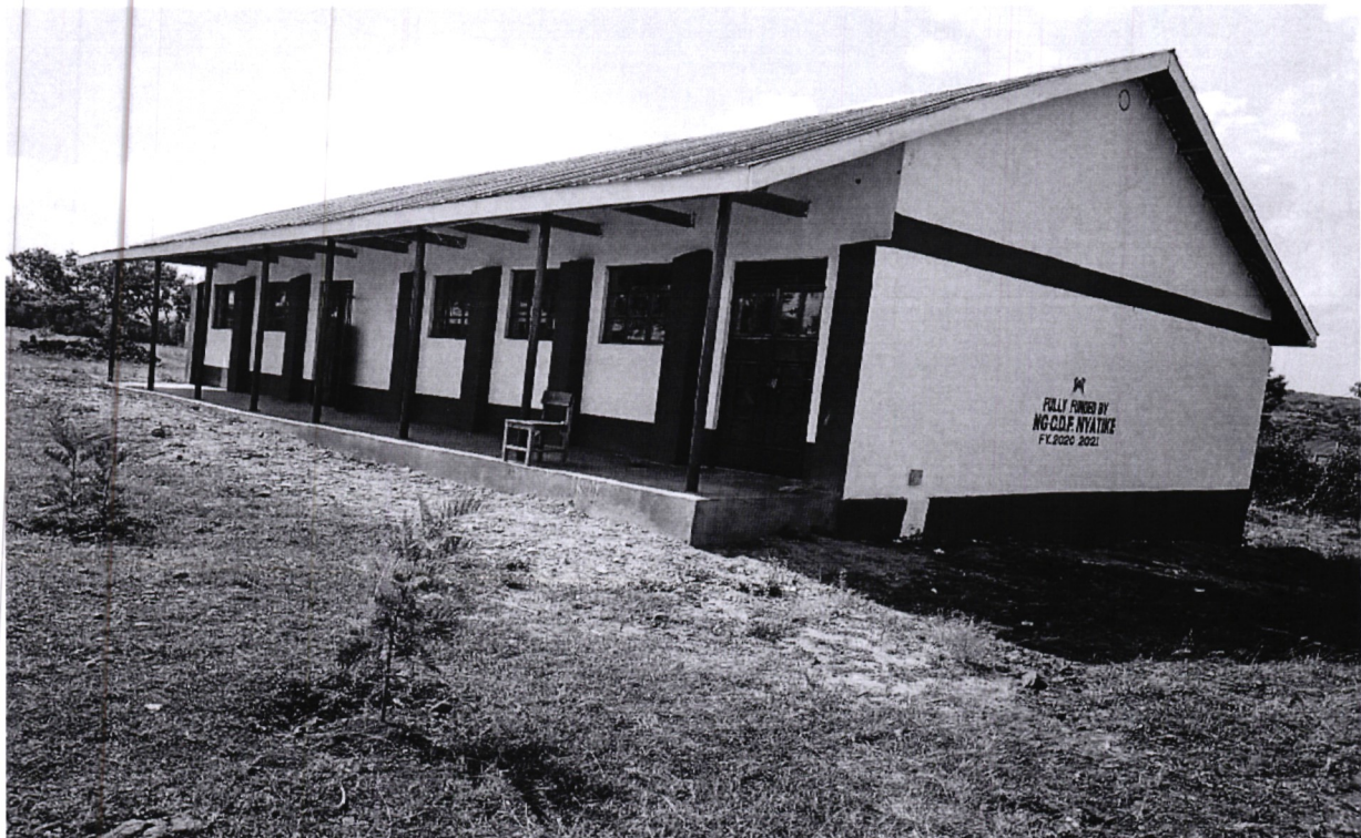
Construction of 2 classrooms at St Jacobs kolanya secondary school
