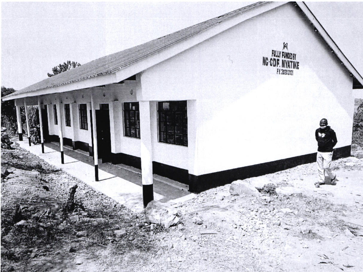
Construction of 2 classrooms at Sidika secondary School
