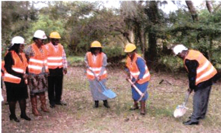
Prof Imbuga (second right) leads the groundbreaking session to pave way for the construction of the laboratory
