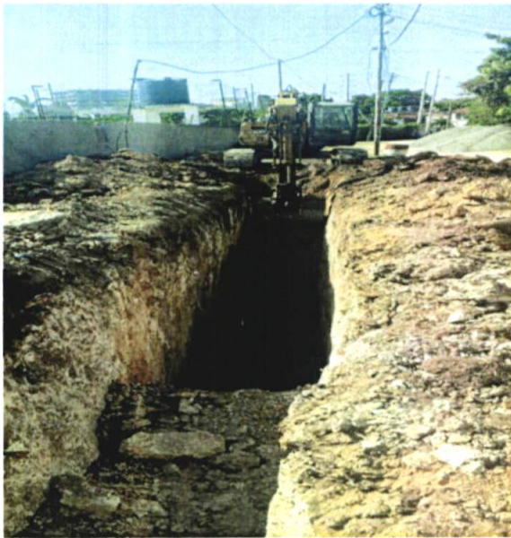
Kilima Road 2,5 Km Sub-Surface Drain
