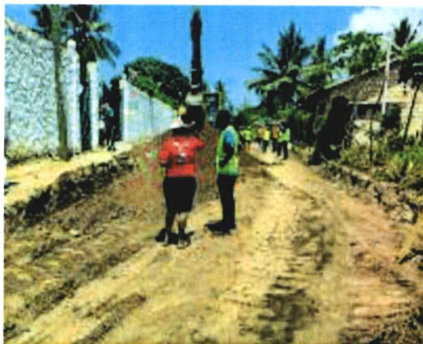
Majaoni Road Preparations
