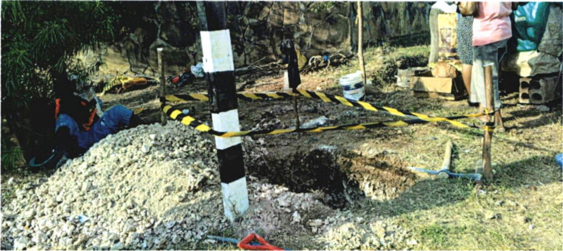
Placement of Reinforcement for Column
