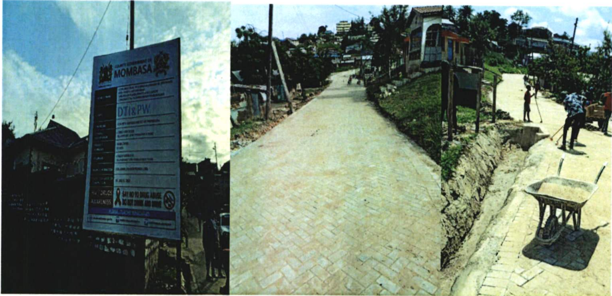
Jitengeni Kwa Thoya Access Road Mikindani ward, Jomvu Sub-county.
