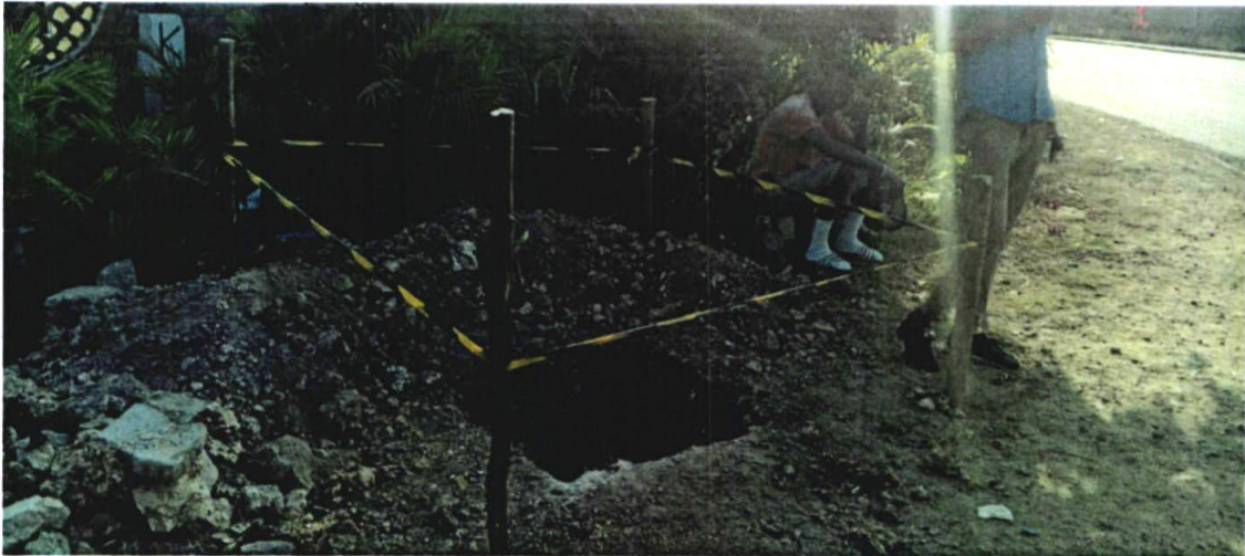
Blinding of the Column Bases
