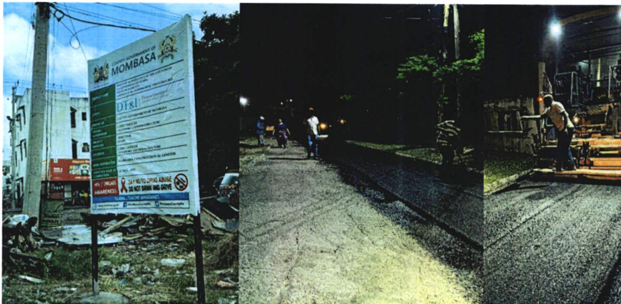
Routine maintenance of Mikanjuni Road Ganjoni/Shimanzi ward, Mvita Sub- County.
