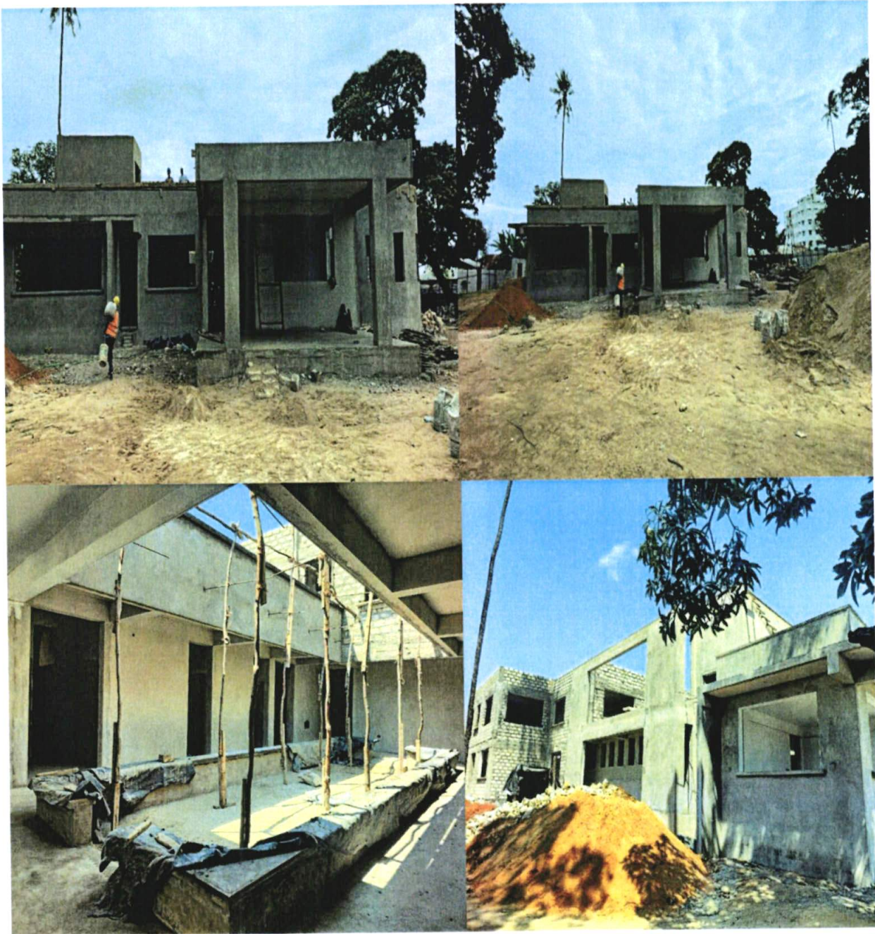
Proposed Level 3 Mjambere Hospital-Work done: 50%
