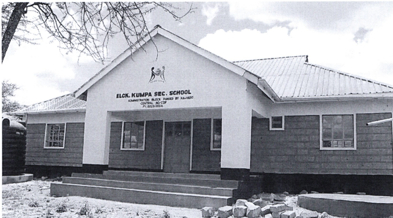
Fig. 1.2 Kumpa Secondary School Administration Block
