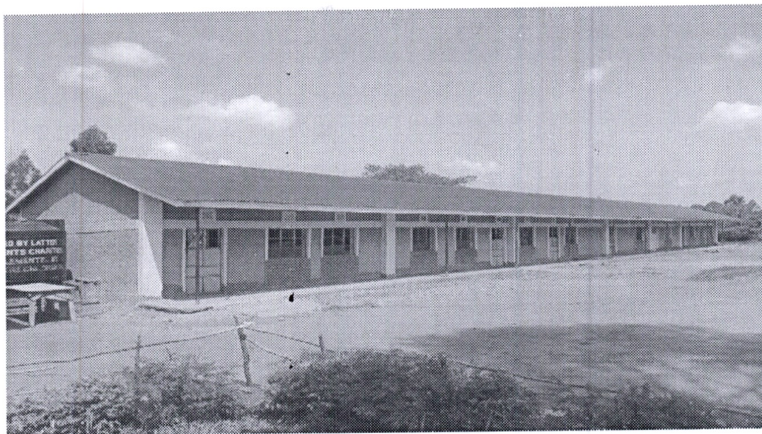
Renovation of four classrooms at Butunyi Primary School
