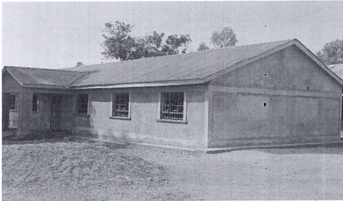
Construction of administration Block at Bulanda Primary School
