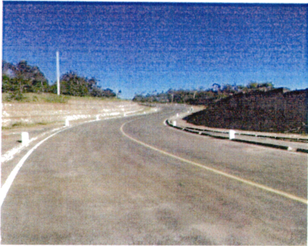
Rd 1 – Kakamega - Ilesi Cleaned and maintained
