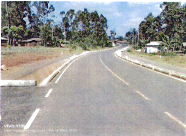
Road 2: Kakamega-Lutonyi Cleaned and maintained
