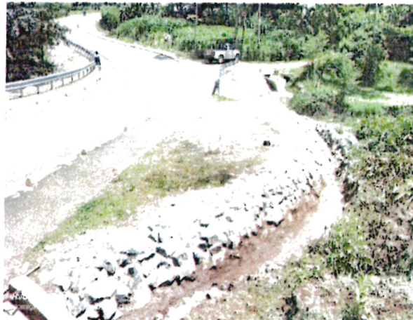
Road 2: Kakamega-Lutonyi Cleaned and Maintained
